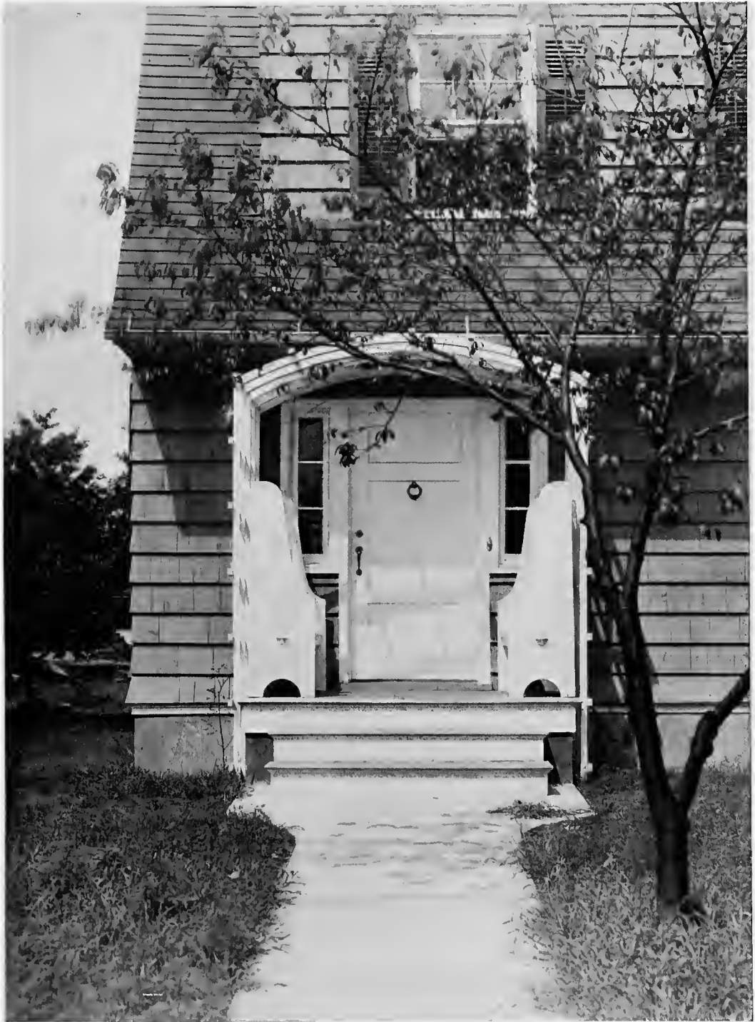
The house as built has widely spaced shingles stained silvery grey, with the outside woodwork white, excepting the second-story shutters which are green
